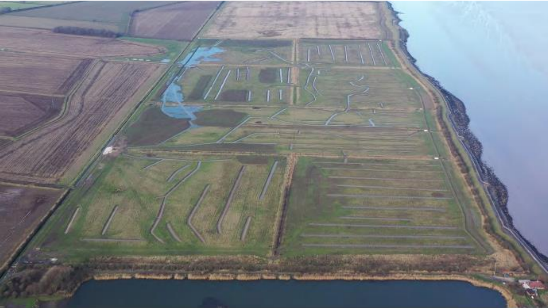
Figure 3. Aerial view of completed HMWG
